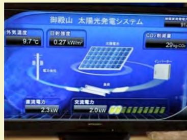
Solar power generation monitor
