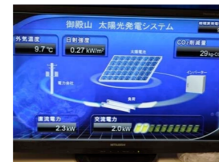
Solar power generation monitor
