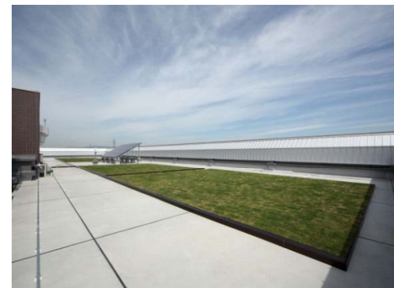
INTEC Manyo Square: Rooftop garden, solar panels
